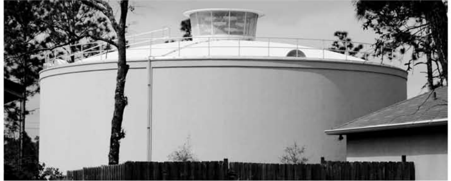
CITY OF DELTONA 1.0 MG WATER STORAGE TANK WITH 2600 GPM AERATOR CONSULTING ENGINEERS: TETRA TECH
